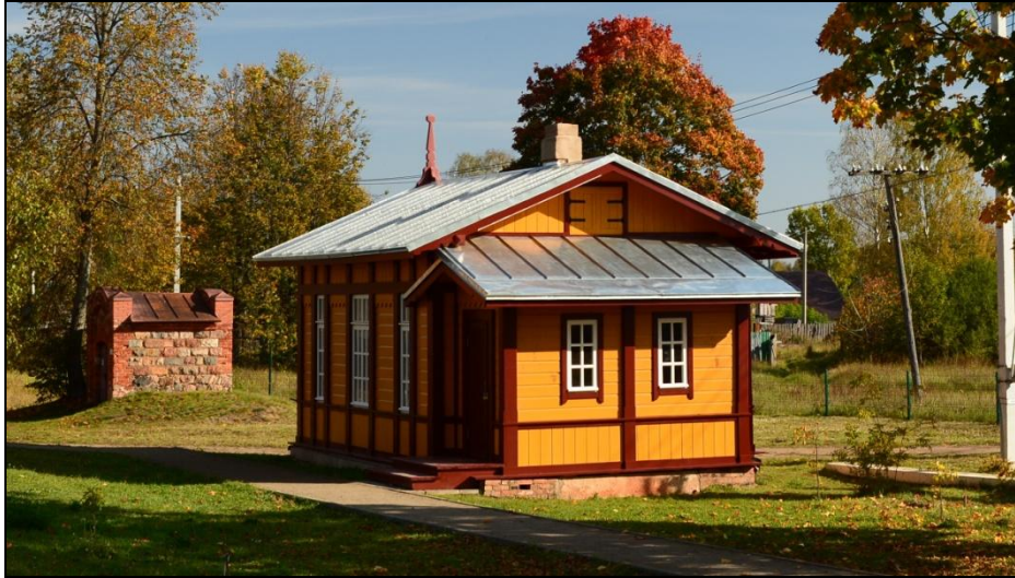
Restored guards' house
