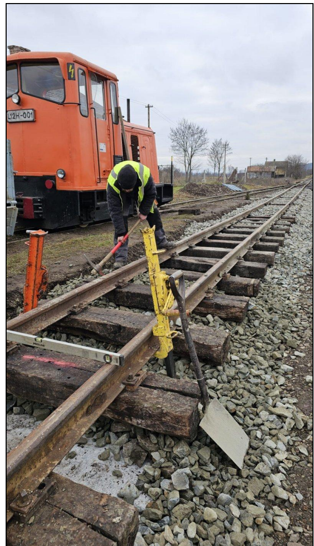
Shovel packing the main line. December 13, 2024
