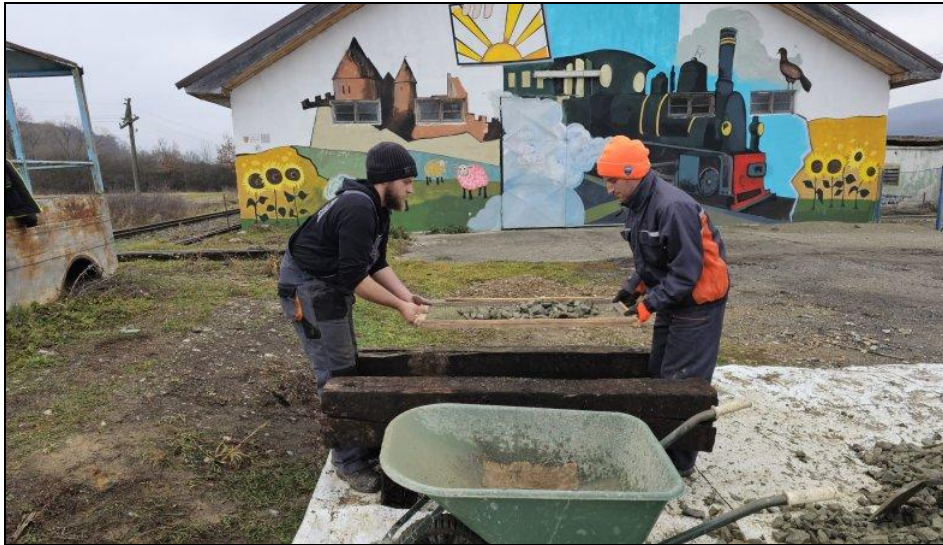
Ballast cleaning in action. December 13, 2024
